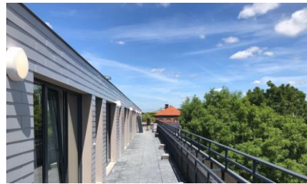
Balcony after conversion
